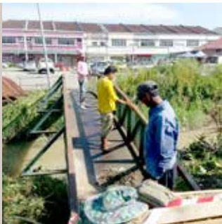
Brushing and painting works on a public steel bridge
