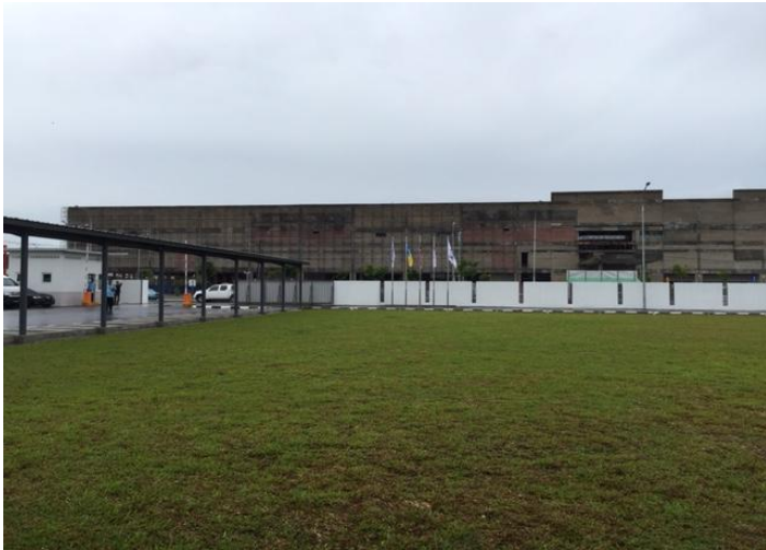
Figure 10: Construction of shopping mall is still ongoing
