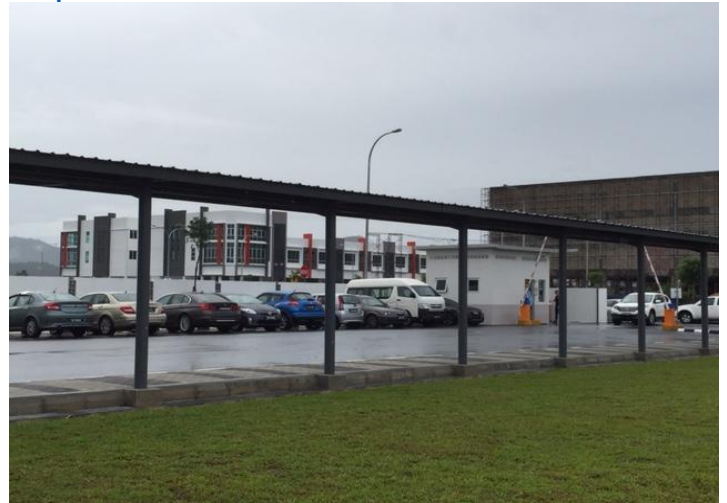
Figure 11: Pearl Avenue (Phase 1) shop lots are almost completed
