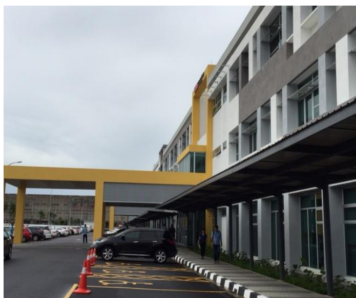
Figure 2: The façade of GEMS International School
