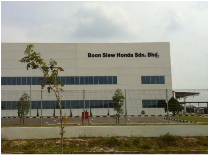
Figure 3 The completed Boon Siew Honda plant at Batu Kawan industrial site
