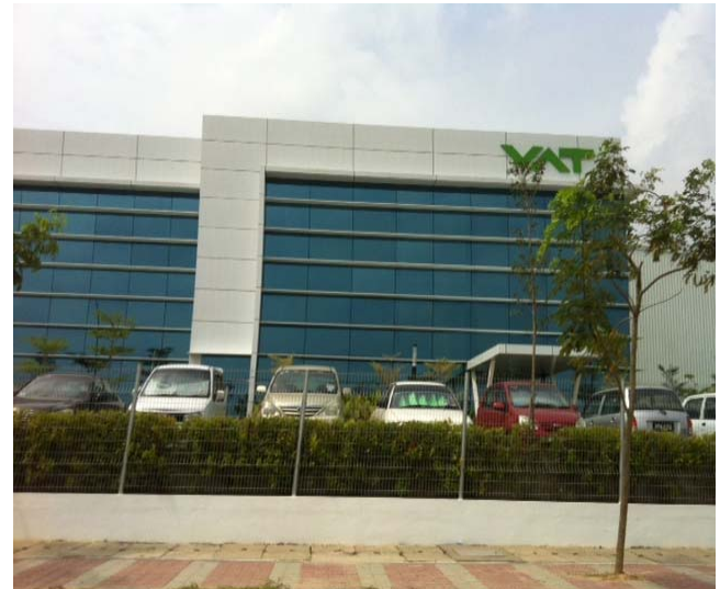
Figure 4 The new VAT plant at Batu Kawan industrial site
