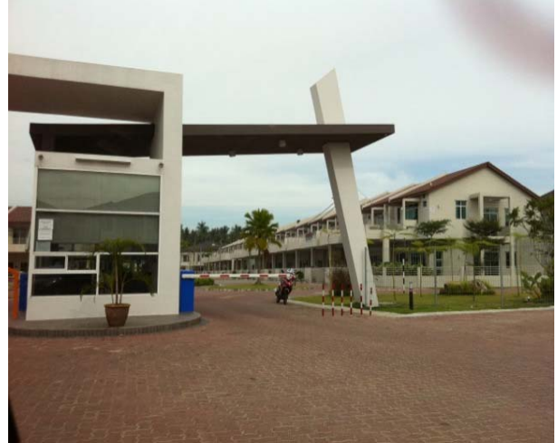
Fig 7: Entrance at the guard house
