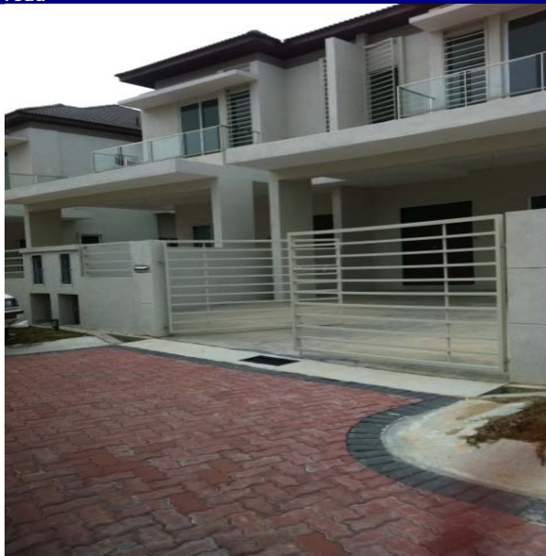
Fig 8: Interlocking concrete pavers are used instead of tar road
