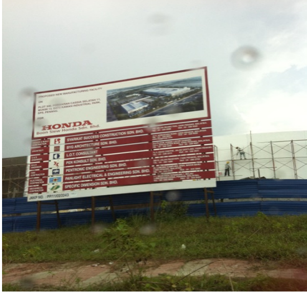
Fig 1: Honda's sign board set up on the construction site
