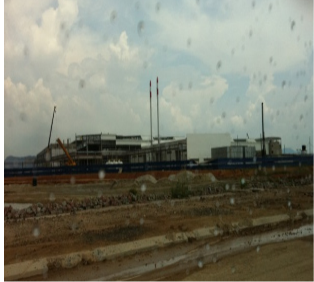
Fig 2: The Hondo plant under construction
